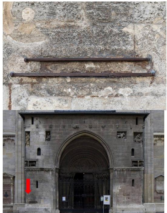
The pictures on the right shows the Vienna Standard length measurements - they are iron bars set into the outside wall of Stephansdom in Vienna, to the left of the big west doors (and red-arrowed in the lower photo). The ends of the bars protrude forwards, creating a **L** shaped space, and measuring rods had to fit exactly into it. The round mark on the wall above them used to be the Vienna Standard Bread Measure - bakers whose loaves were too small were ceremonially ducked in the Danube.
